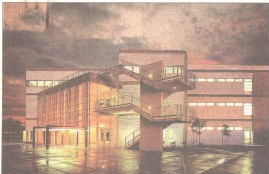
THE ART CENTER employs Ehrlich's bold design that's somewhat of a departure for the rest of the campus. Richard Neutra designed some of the older buildings • Photo: Adrian Velicescu
